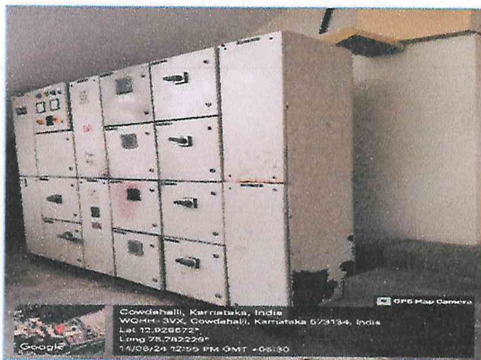
AC DISTRIBUTION WITH MEETRNG CUBICAL BOX
